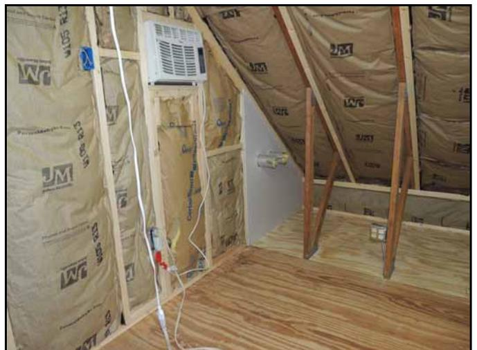
I installed the small wall section of sheetrock so that I could cut out the interior vent openings and finish installing them including the exterior vent covers in the stairwell.
