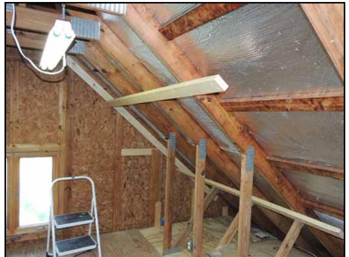
The floor voids have been filled and the outer wall framing is being set in place. The boards nailed into the trusses set the upper position for the wall frame.
