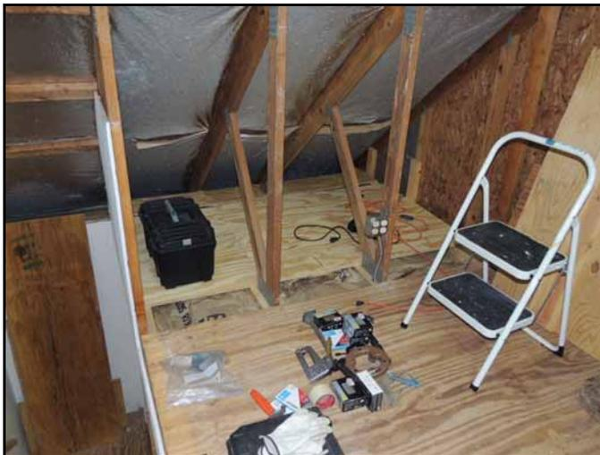
All the flooring is now installed except for the small areas between the trusses. Small lengths of wood were screwed into the trusses to act as nailing lips for the small sections of flooring that will fill these small floor voids.
