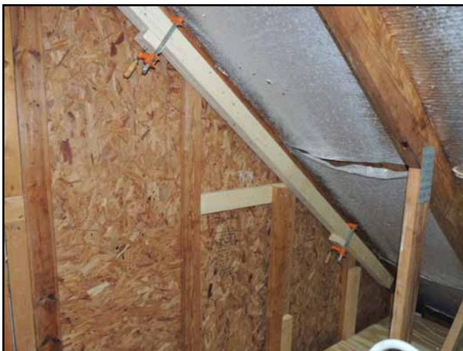
I used a lot of clamps to set the framing in place and then pre-drilled holes for wood screws. For this entire project heavy duty wood deck screws were used.
