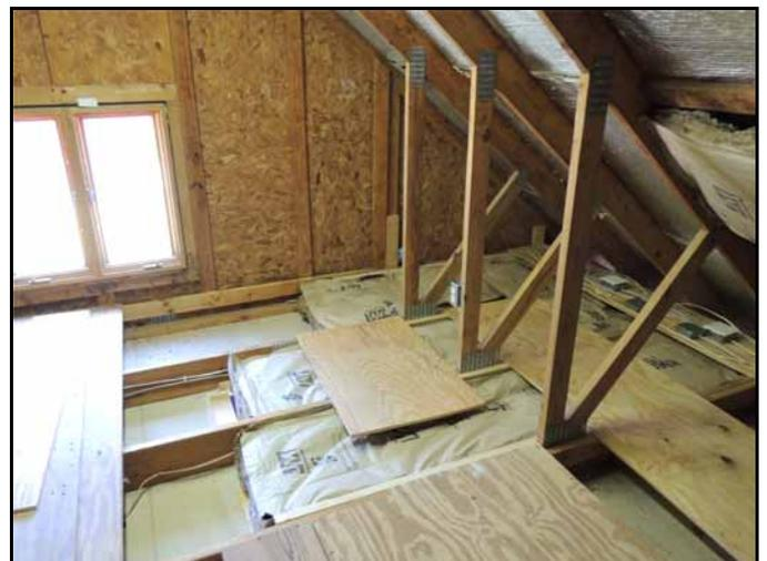
Insulation was added to the floor between the trusses and as it was installed, the flooring was positioned so that it could be screwed down. Screw holes were pre-drilled and beveled so that the wood screws would sit flush.
