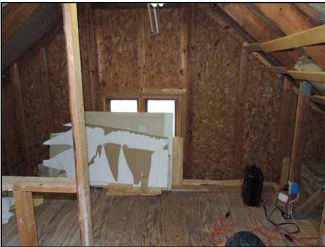
The area that will be the clean room will be large, but first the electrical wiring has to be moved and new outlets installed. The framing needs to be installed for the walls and the entire area are needs to be insulated.
