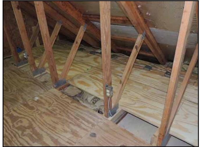
Additional flooring was added between the truss braces. These smaller areas will be storage for kits and supplies.
