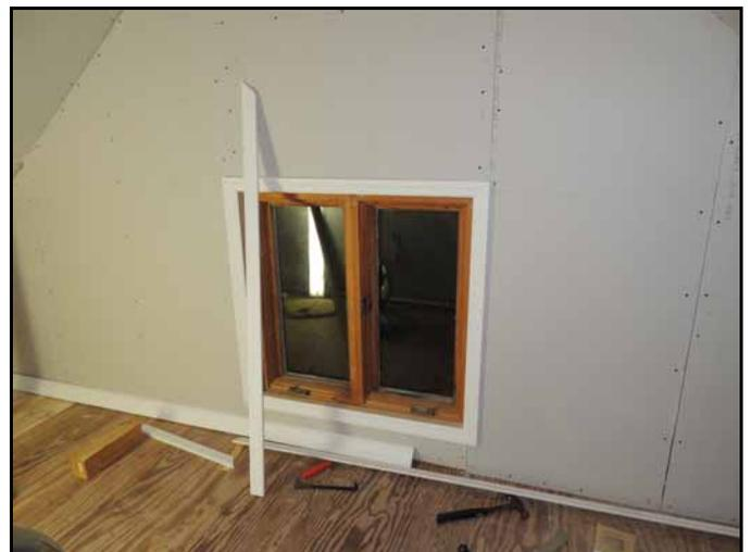
Once all the sheetrock was installed the window was framed out and then wood trim was added to the floors and around the door.
