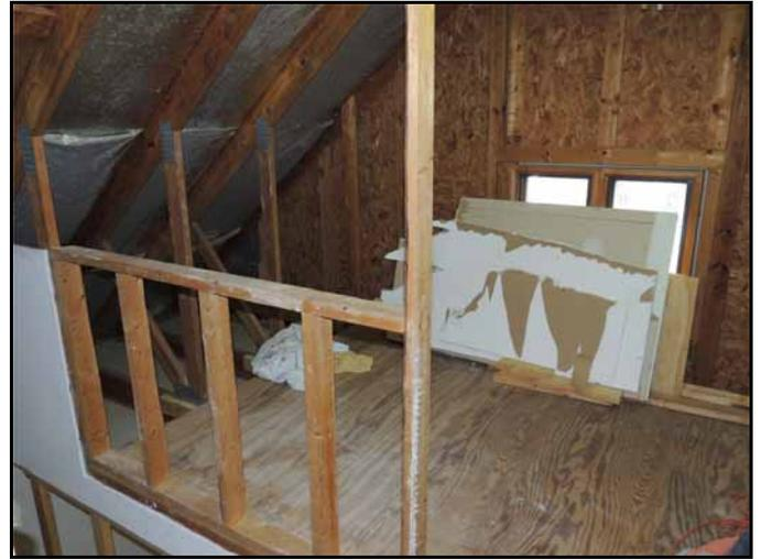
This area will be the clean room for airbrushing. I plan to have dual exhaust ventilators and a separate wall air Conditioner. The sheetrock and the existing framing is being removed so that I can pull the floor.
