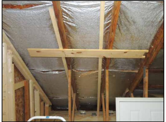
Each truss had an extra length of wood attached so that there would be a 3 inch surface for connecting sections of sheetrock. Since I was doing all the interior sheetrock work myself, I would need to install small sections at a time.
