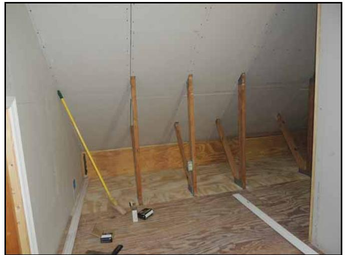
Since the small walls at the bases of the trusses were designed to allow access to the electrical splice boxes these areas were covered with 1/2 inch plywood.
