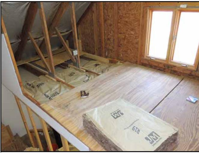
The insulation is almost complete and the flooring is set in place and some of it has been screwed down.
