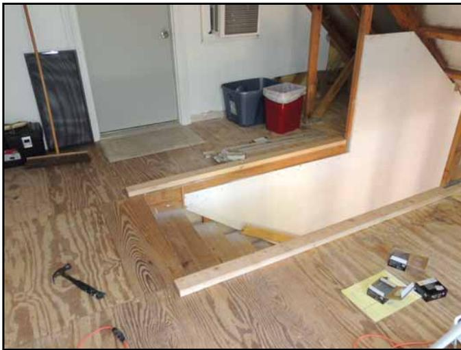
The floor studs for the stairwell walls and the door frame were carefully measured and marked on the floor and then sections of wood were screwed into the floor.
