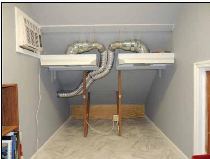
The ventilators have been installed along with the flexible piping.
