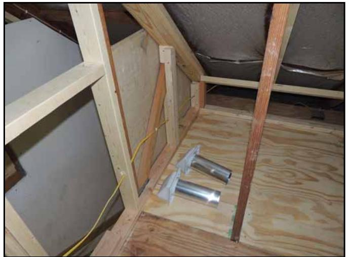
The dual vents for the clean room were measured and then traced onto the sheetrock and then cutouts were made for the piping.
