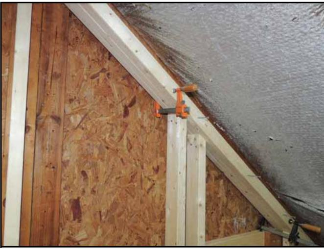
A nailing lip needed to be added to the outer wall frame for the sheetrock. I like to have at least a 1.5 inch nailing lip.
