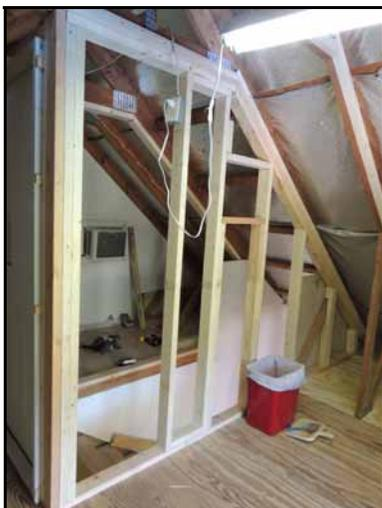
One side of the stairwell wall frame has been completed and additional studs and cross members will need to be added. Once all the framing is complete the electrical work will be done.
