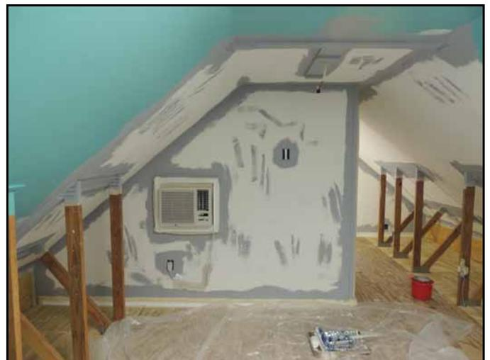
The surfaces were primed and then finished paint was applied around the edges to box in areas that will be rolled.
