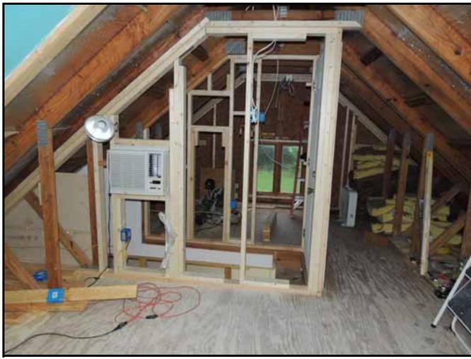
The stairwell wall which will hold the large air conditioner which is also a heater is just about complete.
