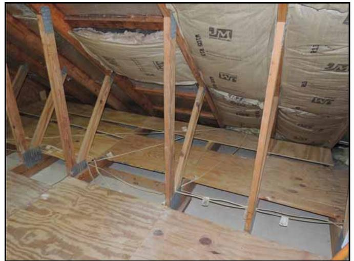
There was a lot of wiring that needed to be moved. Every wire was traced and then tagged, with what plug, switch or light it provided power to. Each wire will need to be spliced and lengthened.
