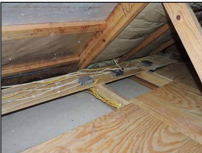
A separate platform was installed just for the wiring and splice boxes. Each wire was labeled and each splice box was also labeled so that it would be easy to determine where wires were located should the need arise.
