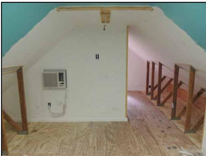
The seams were covered with fiberglass screening and then filled with wall mud. After the seam mud dried I plastered the walls.
